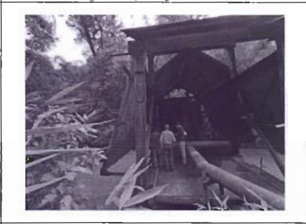
Fig:19 Pump house beside Lunar river
